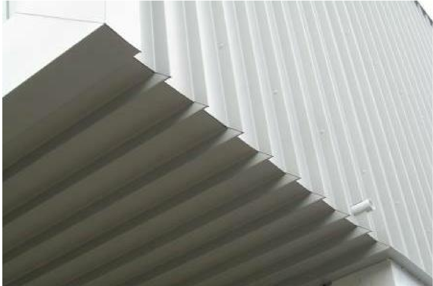
MRS1: METAL ROOF CLADDING - LIGHT COLOUR
